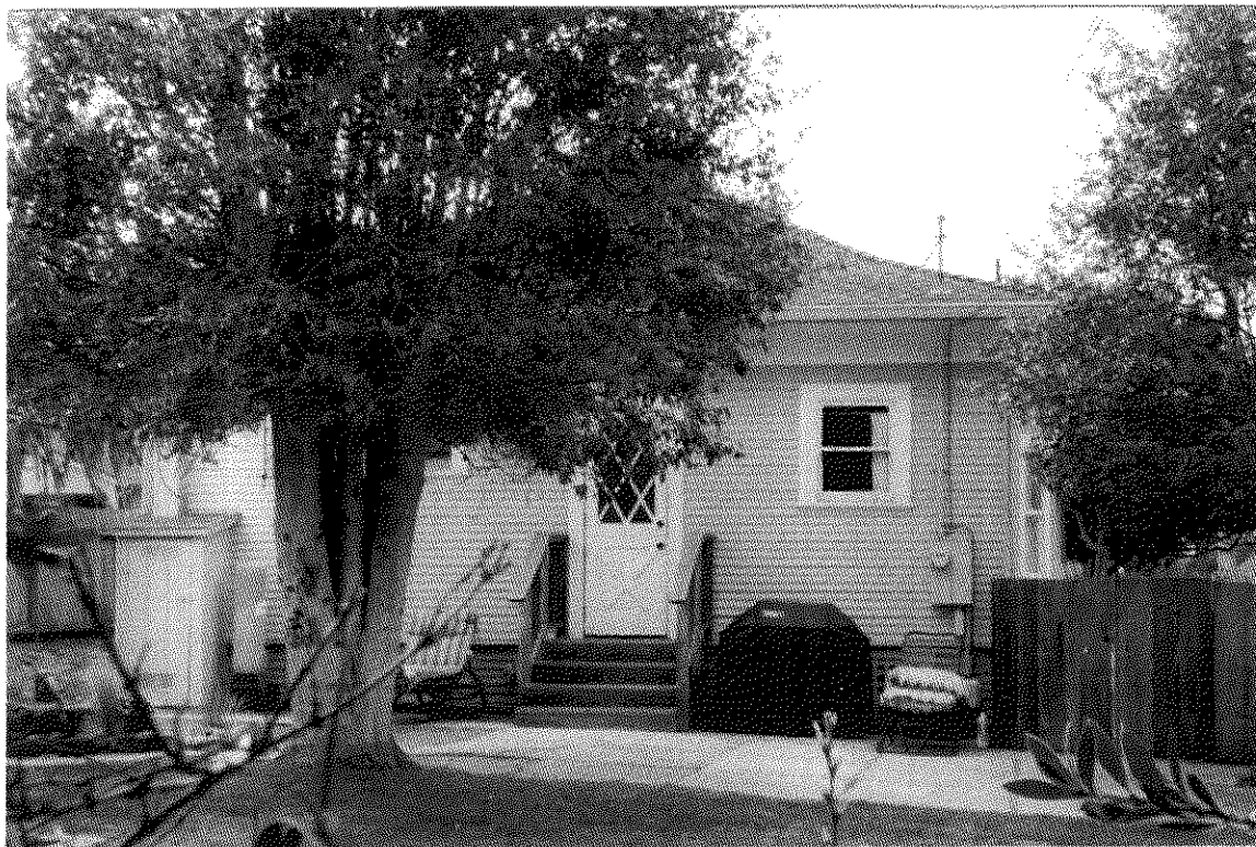
Photo #5. Looking west at the rear (east) elevation, note fenestration changes from c. 1912. April, 2015.
