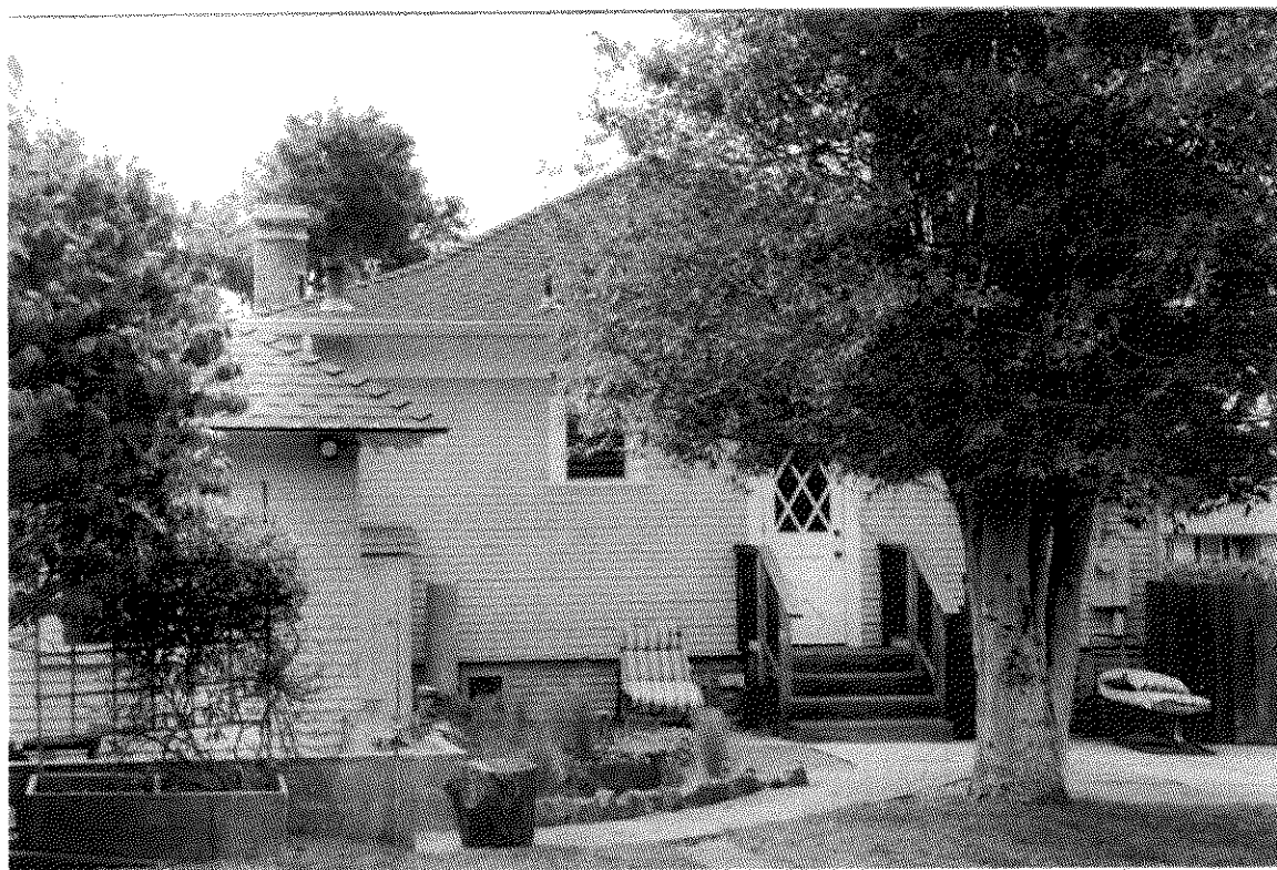
Photo #6. Looking west at the rear (east) elevation, note small window for proposed reuse, April, 2015.
