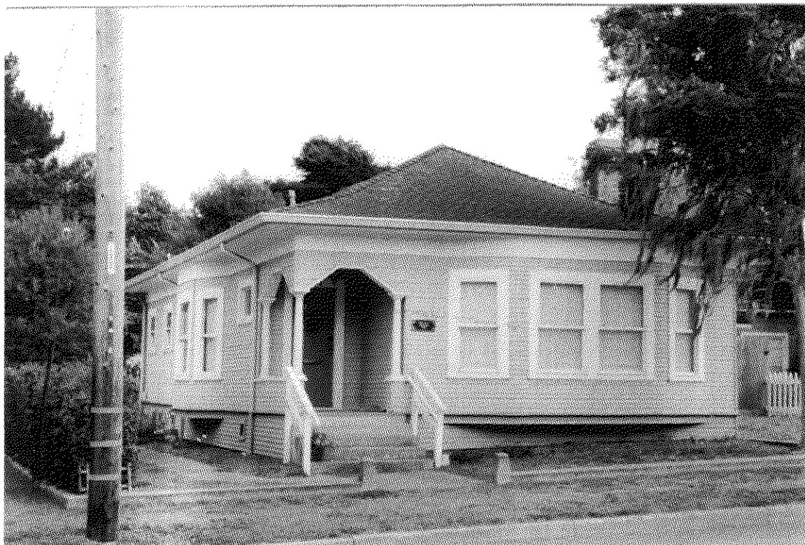
Photo #2. Looking SE at the west facing facade & north side-elevation, April, 2015.
