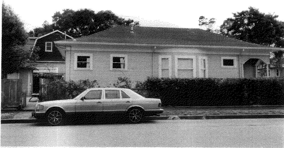
Photo #3. Looking south at the north side-elevation, April, 2015.
